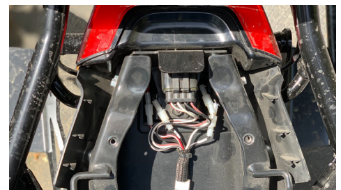
Figure 17. Wires Inside Tail Frame
